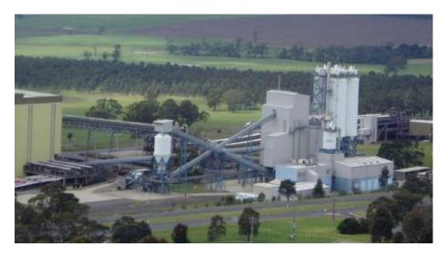
Figure 23: Steam fluidized bed drying plant, Loy Yang (Allardice 2015)
