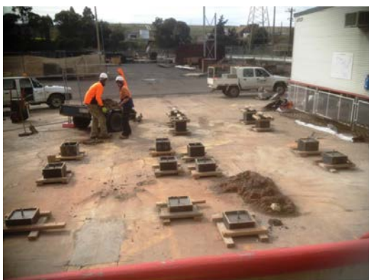
Figure 3C: Civil construction at site.
