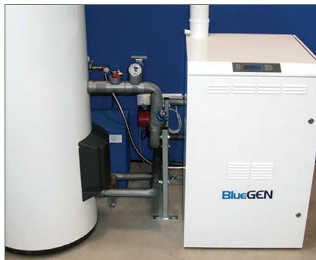
Figure 74: BlueGen® converts natural gas into electricity
