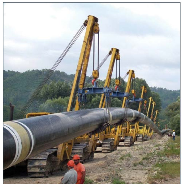
Figure 59: A CO 2 pipeline being laid in the US
