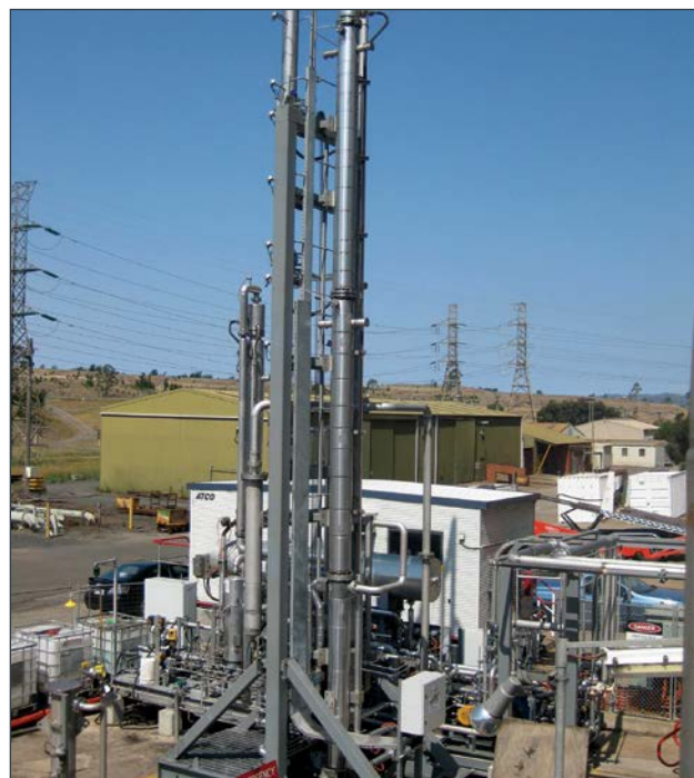
Figure 44: UNO MK 3 pilot plant at Hazelwood
