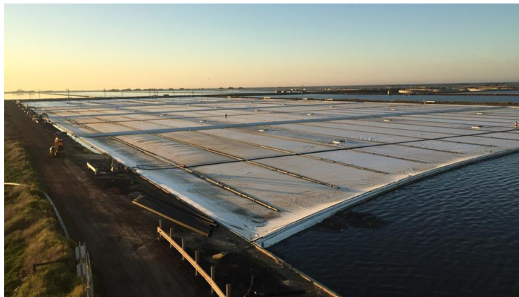
Figure 17: Melbourne Water's Western Treatment Plant in Werribee 29
