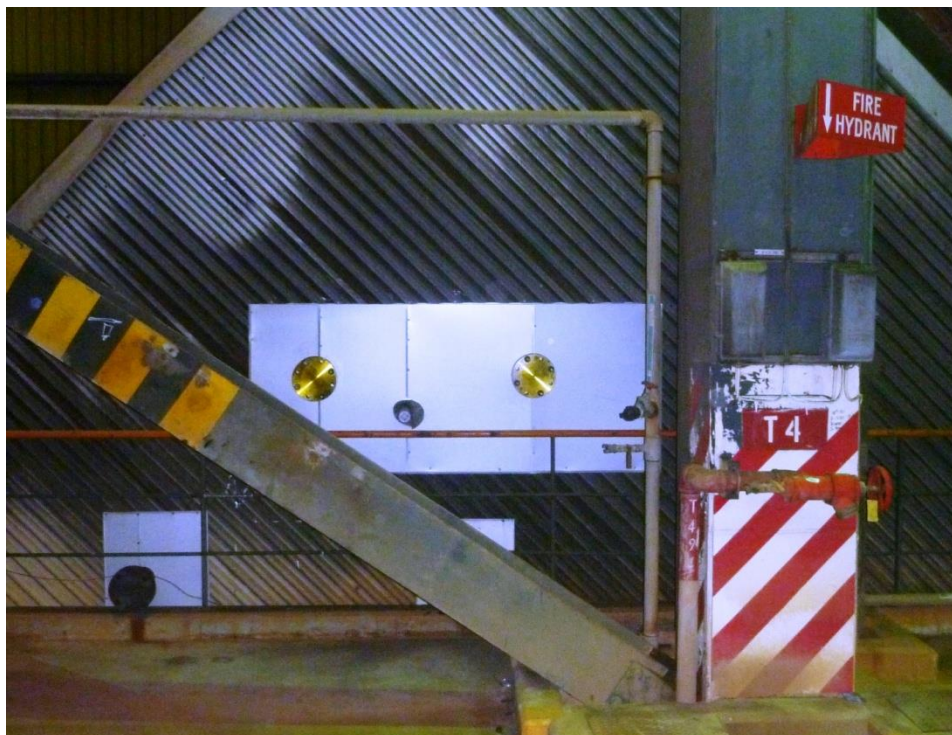
Figure 15 - Completed Port Installation
